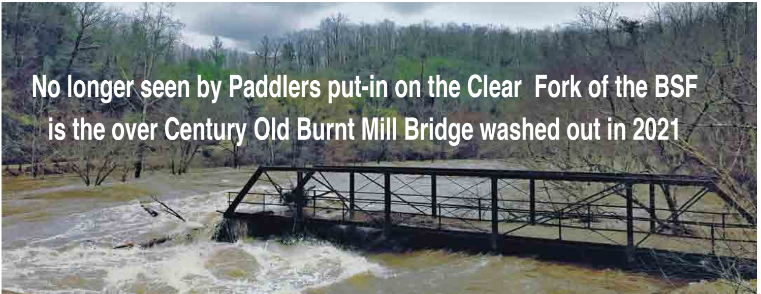
What's pictured in this photo isn't as significant as what isn't pictured, after flood waters swept away the eastern half of the historic Burnt Mill Bridge over Clear Fork River near Robbins | Photo: Nancy Chambers
